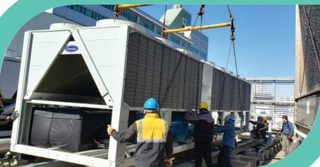
4. Replacement work of a new set of air-cooled chillers
