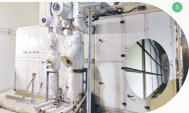
1. Deploying nano-technology low energy, high-efficiency air filter system to improve IAQ performance
